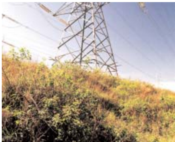
Lantana in powerline easement.
